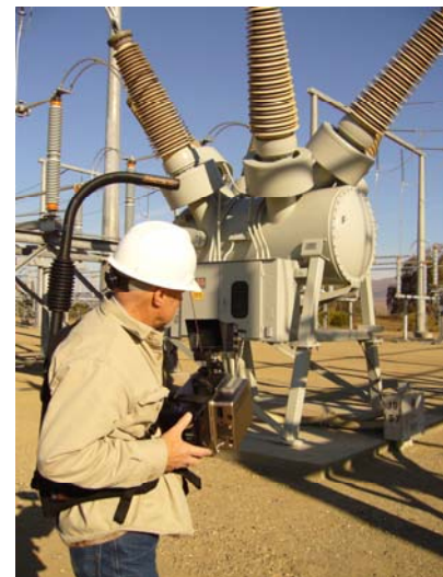
Figure 4. Sherlock shown with an operator looking for leaks at a substation.
